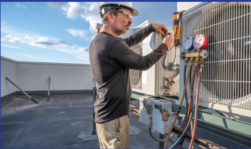
HVAC SYSTEM MAINTENANCE
