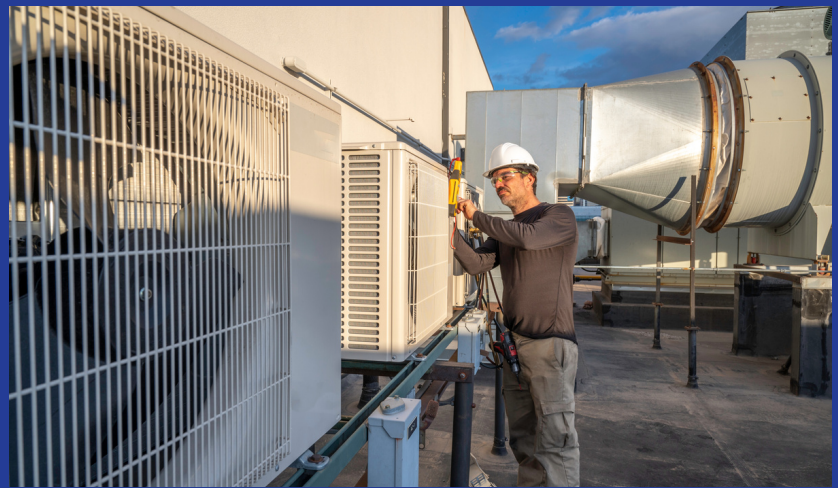
HVAC SYSTEM REPAIR
